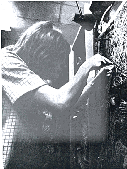
Skilled hand-wiring goes into Control Data's 7600 computers at Chippewa Lab.
